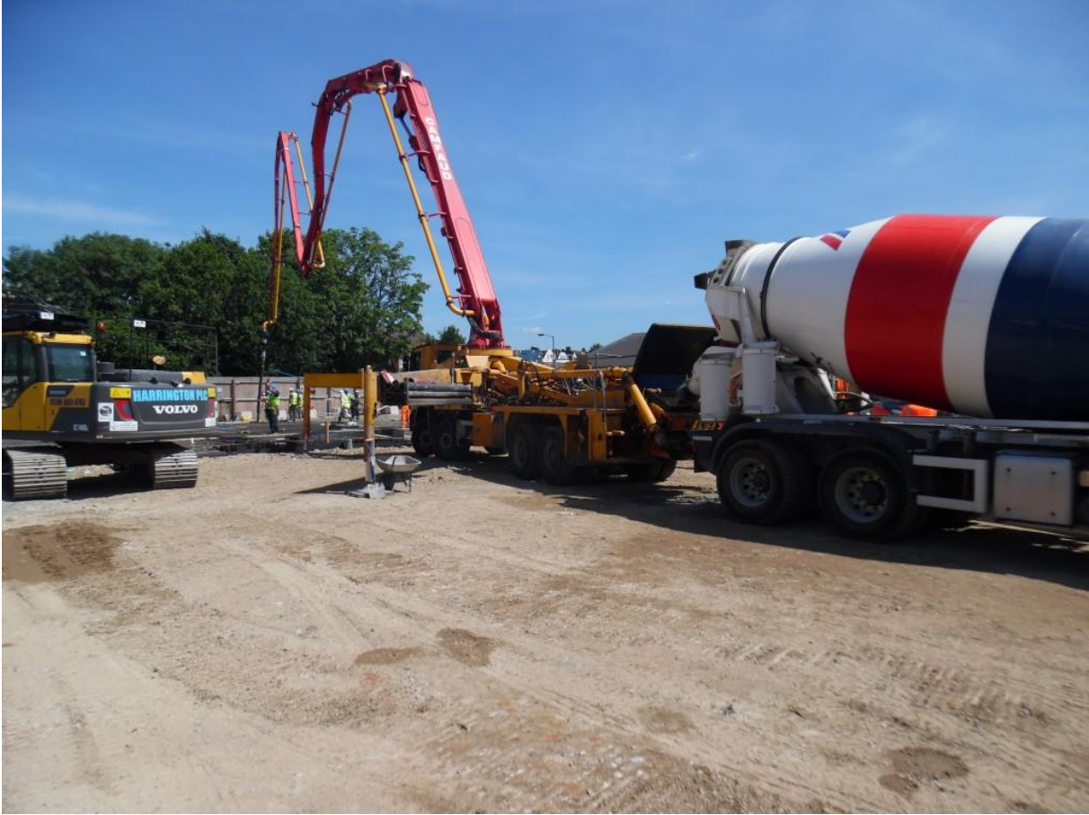
Image 01, 07-07-2017; concrete pump setup Friday morning 07-07-2017; concrete lorries filling hopper
